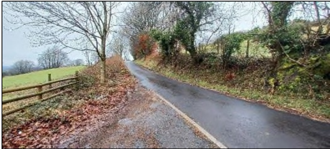
Photograph 3.2 Site access visibility to the north
